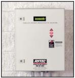
NXT Quick-Set Repair Permits the operator to reset the door using the System 3 controller after aligning the bottom bar.
